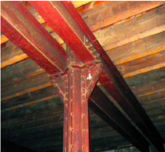
Image 3: 4th floor ceiling
